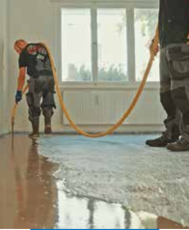
Application of Ultraplan Xtra with a pump
