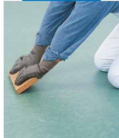
Massaging of linoleum joint
