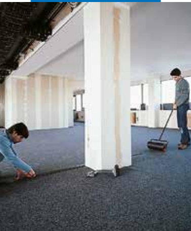
Pressing carpet joint with roller
