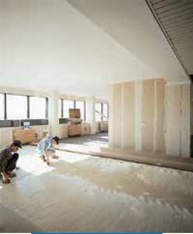
Installing large-size sheets with Aquacol T
