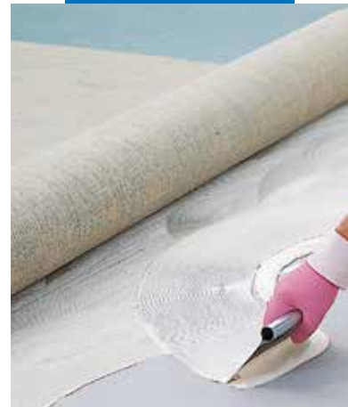
Installing linoleum with Aquacol T
