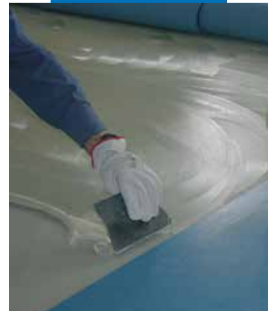
Application of Ultrabond Eco V4SP - San Martino Rest Home - Italy
