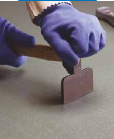
Pressing down the junction between sheets
