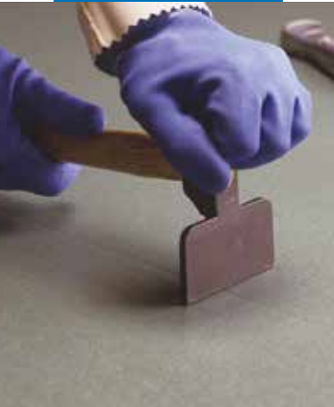
Pressing down the junction between sheets
