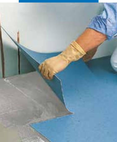
Laying conductive PVC tiles with Ultrabond Eco V4 SP Conductive
