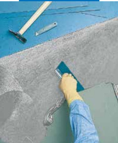
Spreading Ultrabond Eco V4 SP Conductive
