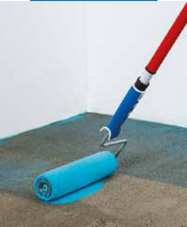
First coat application of Mapeproof Primer
