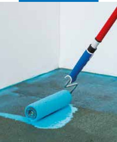
Second coat application of Mapeproof Primer
