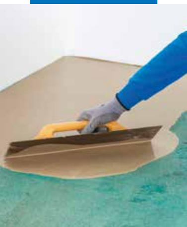
Self-levelling compound application on Mapeproof Primer
