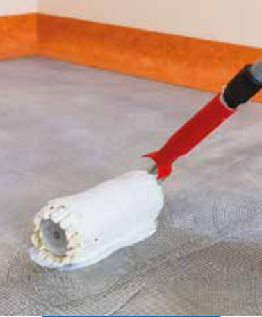
Application of Eco Prim T with a roller
