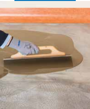
Spreading Ultraplan Fast Track with a metal trowel
