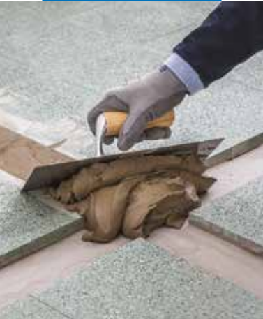
Filling a cable run with Planipatch Fast Track
