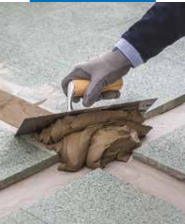
Filling a cable run with Planipatch Xtra
