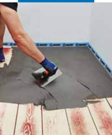
Application of Planipatch Xtra + Latex Plus on wooden substrate
