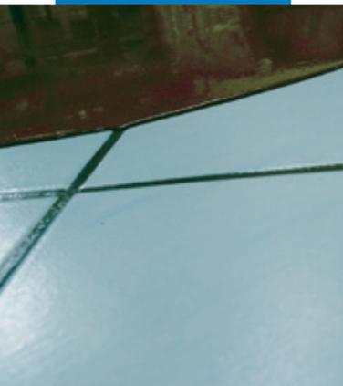
Detail of the application of **Ultraplan** on an existing ceramic tile floor after the application of **Eco Prim T Plus**
