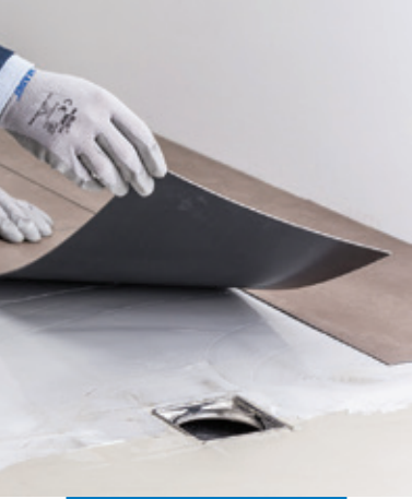
Application of LVT floorings with Ultrabond Eco MS 4 LVT in damp surroundings
