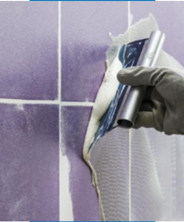
Spreading Ultrabond Eco MS 4 LVT Wall with a notched trowel on a non-absorbent substrate
