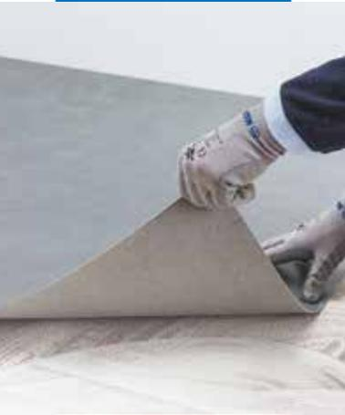
Bonding rubber flooring on a non-porous substrate with Ultrabond Eco S1000 1K
