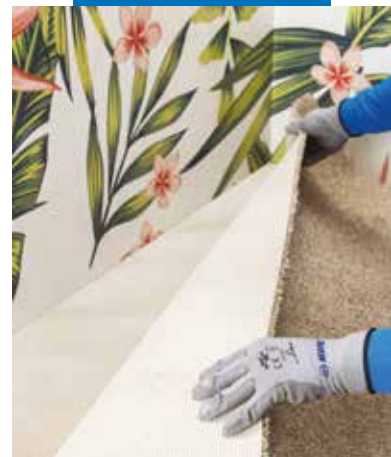
Broadloom carpet installation onto the acoustic underlay (double stick installation)
