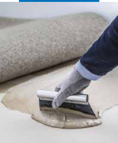
Application of Ultrabond Eco TX3 for installing needle-felt
