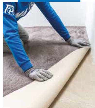
Action Back® backed broadloom carpet installation
