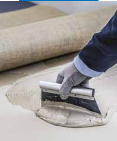
Application of Ultrabond Eco TX3 for installing linoleum
