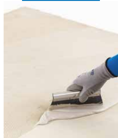
Ultrabond Eco TX3 application onto self-levelling compound (direct stick installation)
