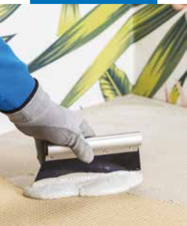
Ultrabond Eco TX3 application onto the acoustic underlay
