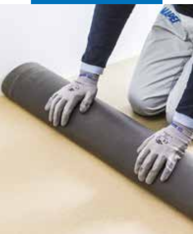
Acoustic underlay installation
