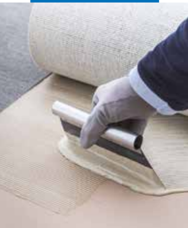
Action Back® backed broadloom carpet installation
