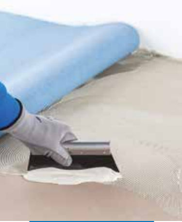
Ultrabond Eco TX1 application
