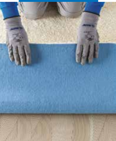
Felt backed broadloom carpet installation
