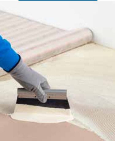
Ultrabond Eco TX2 application
