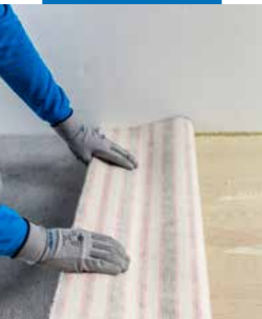
Broadloom carpet installation
