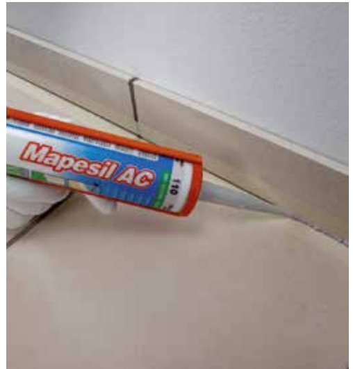
Seal the gap between the skirting board and the floor with a suitable flexible sealant from the Mapei range
