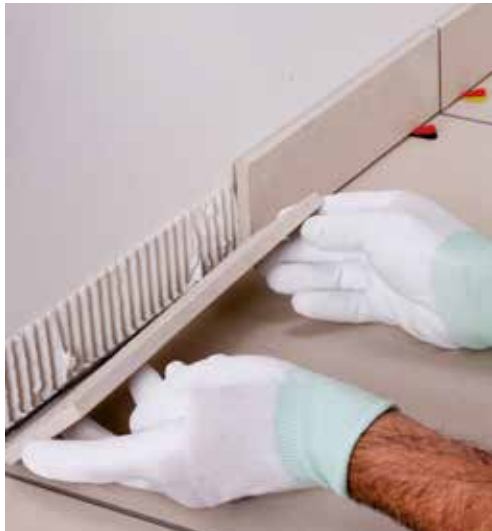
Apply the skirting around the room without letting it come into direct contact with the floor
