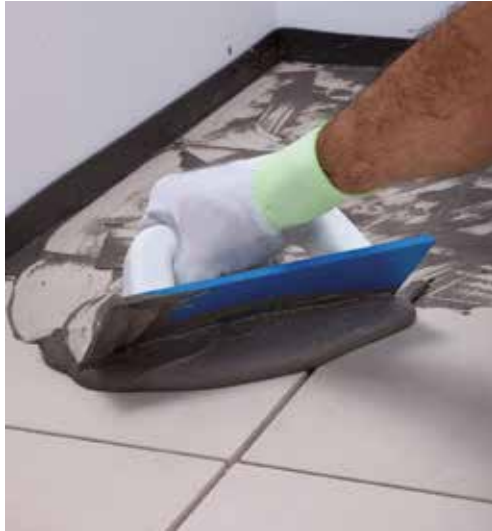
Grout the surface of the room
