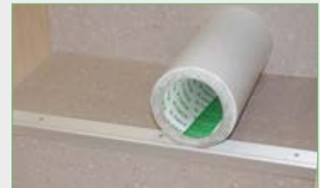
Full area CV-covering that is applied on primed stairs
