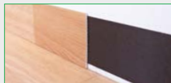
Installation of profiles made of CV / heterogeneous PVC
