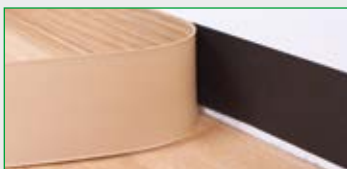
Installation of PVC-soft-skirting
