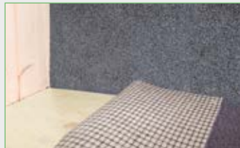
Installing the textile covering onto the area covered with Step-FLOOR
