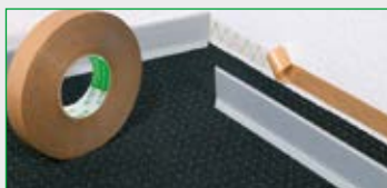
Installation of a solidcore-skirting profile
