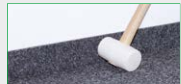
Applying pressure to a freshly installed needle-felt strip
