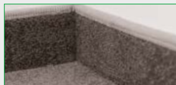
Installation of textile skirting strips
