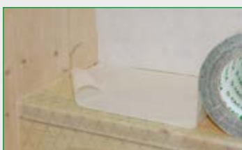
Full area application of the adhesive tape
