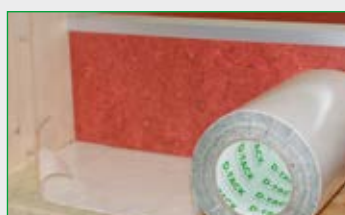
Installation of a linoleum covering
