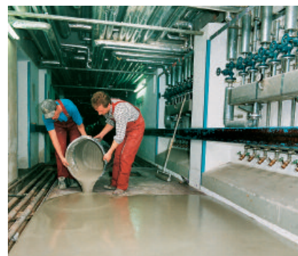
PCI Zemtec 1K self-levelling floor leveller for direct use applied over the entire area.
