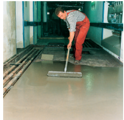
PCI Zemtec 1K, poured and spread on to the tack-free, cured primer, levelled and de-aerated with a spiked roller during the application.
