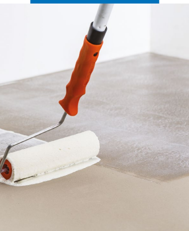
Ultrabond Eco TX3 application for fixing an acoustic underlay
