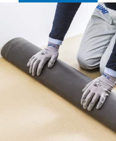
Acoustic underlay installation
